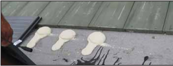
Polyfoam installations are also recommended for high wind applications.
